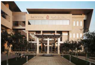
RAK HOSPITAL, DUBAI
